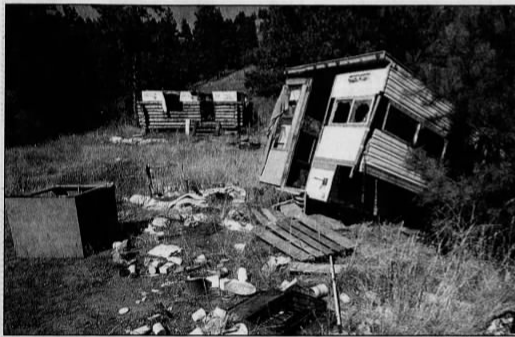
TOP RIGHT: A damaged van is one of a number of items Kenneth and Bernadette Chester left behind when they moved out of a subdivision north of Craig sometime during the past two years. ABOVE: A half-finished log cabin, a camper top and a field full of litter are all that's left on the Chesters' former property.
