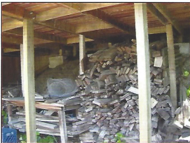
No deck, regardless of the material used to build it, would be safe if this amount of fuel beneath the deck caught fire. Even decks that may have a noncombustible surface, such as concrete, use lumber and timbers for structural support and those materials can catch fire.
